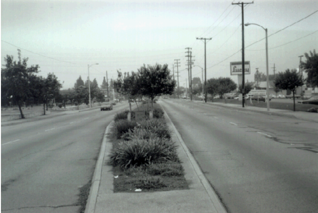
PICTURE 13. VIEW OF AZUSA AVENUE, LOOKING SOUTH TOWARD SAN BERNARDINO ROAD. THE GENERAL PLAN CALLS FOR MAINTAINING THE PHYSICAL AND AESTHETIC CONDITION OF PUBLIC RIGHTS-OF-WAY, WHICH DIRECTLY SUPPORT AND ARE INTERTWINED WITH LAND USE.
