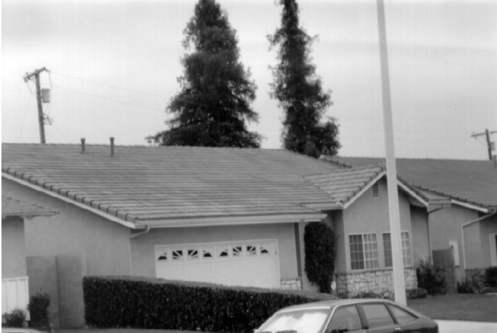
PICTURE 13. CONVENTIONAL MODERN HOME. THE GENERAL PLAN ESTABLISHES AN ADMINISTRATIVE STRUCTURE FOR MAINTAINING FIRE-INHIBITING REQUIREMENTS AND STANDARDS, SUCH AS TILE ROOFS, FOR NEW CONSTRUCTION AND SUBSTANTIAL ADDITIONS.
