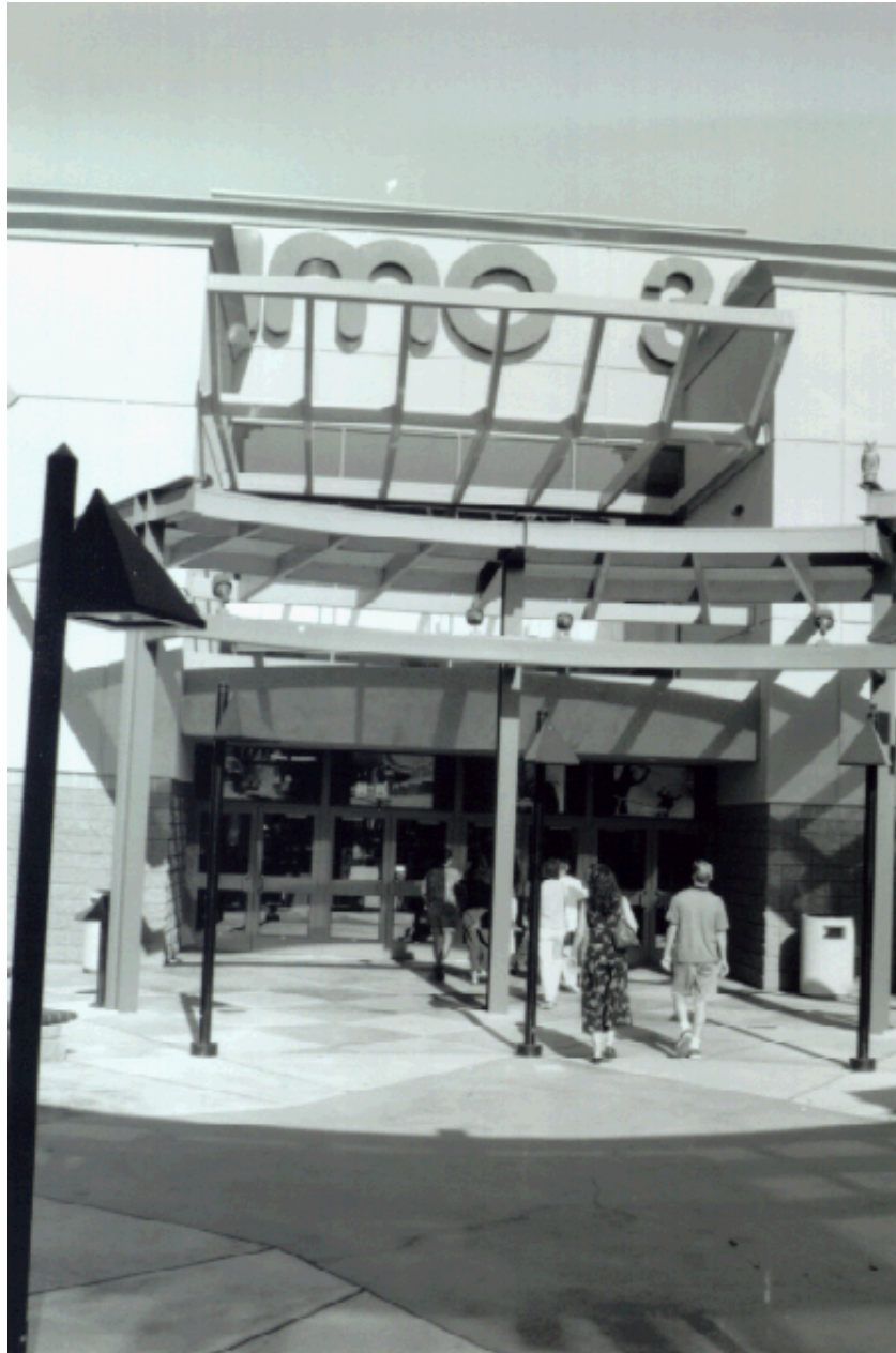
PICTURE 16. AMC 30-PLEX MOVIE THEATRE AT COVINA TOWN SQUARE SHOPPING CENTER, AT AZUSA AVENUE AND ARROW HIGHWAY. THIS AND OTHER VIBRANT COMMERCIAL USES COMPLEMENT COVINA'S HOUSING.
