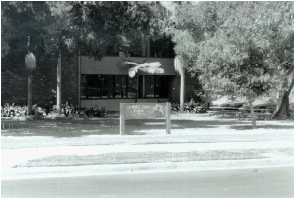
PICTURE 10. THREE OAK PARK IN THE VILLAGE OAKS OFFICE PARK, NEAR HOLT AVENUE AND THE SAN BERNARDINO FREEWAY. LIKE SCHOOLS, LIBRARIES, HOSPITALS, AND OTHER USES, PARKS ARE CLASSIFIED AS NOISE-SENSITIVE UNDER THE GENERAL PLAN PROCESS, A MATTER THAT WILL BE CONSIDERED IN PARTICULAR CONSTRUCTION APPLICATIONS.
