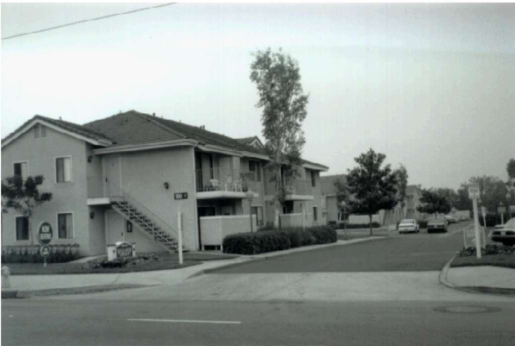
PICTURE 11. VILLAGE GREEN SENIOR CITIZEN APARTMENT COMPLEX, ON COVINA BOULEVARD JUST EAST OF CITRUS AVENUE. VILLAGE GREEN WAS DEVELOPED WITH COVINA REDEVELOPMENT AGENCY ASSISTANCE AND PROVIDES QUALITY HOUSING FOR MANY LOWER INCOME SENIOR HOUSEHOLDS.
