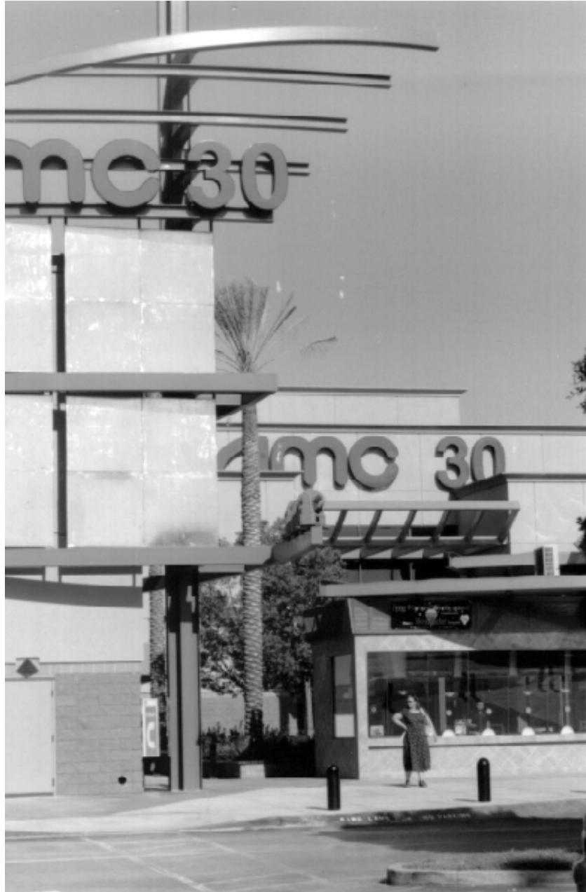
PICTURE 16. THE NEWER AMC 30 MULTI-PLEX MOVIE THEATRE AT THE COVINA TOWN SQUARE SHOPPING CENTER, AT AZUSA AVENUE AND ARROW HIGHWAY. COVINA'S INFRASTRUCTURE MUST SUPPORT MAJOR COMMERCIAL DEVELOPMENTS SUCH AS THIS ONE, WHICH ARE ESSENTIAL FOR MAINTAINING COMMUNITY ECONOMY, IMAGE, AND CHARACTER.
