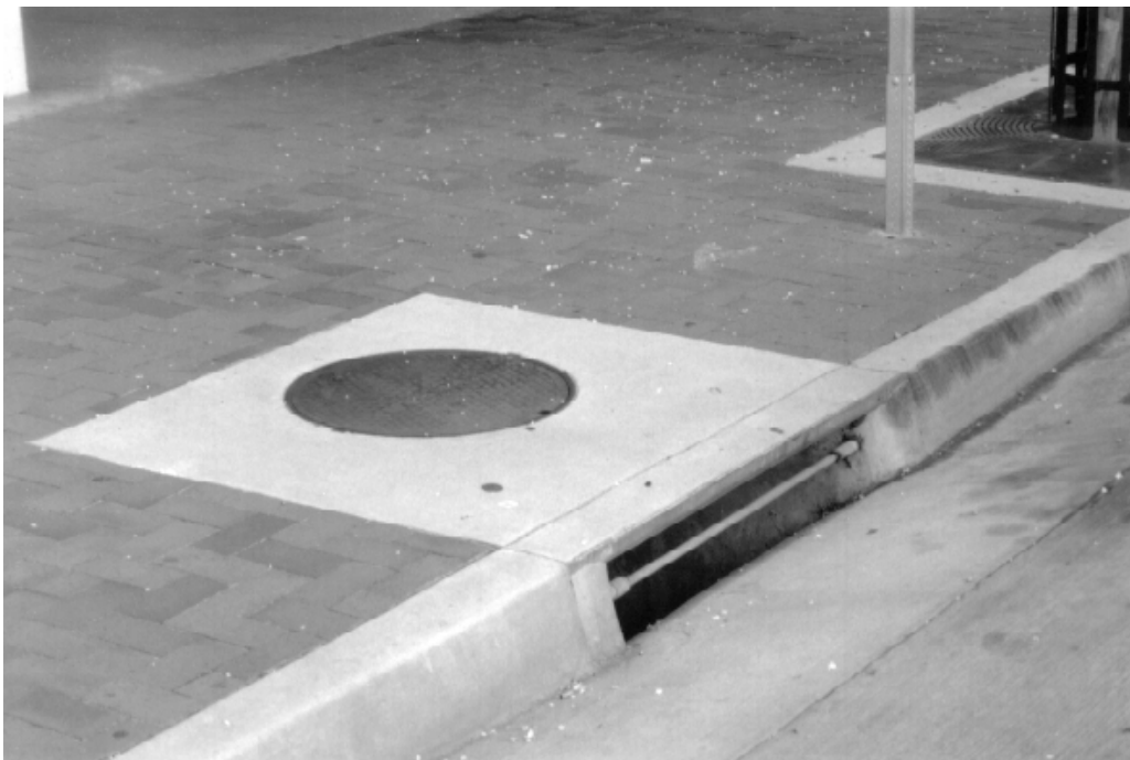
PICTURE 10. TYPICAL STORM DRAIN INLET. BECAUSE OF THE ESSENTIAL FUNCTION THAT IT SERVES, THE GENERAL PLAN ADVOCATES MAINTAINING AND, WHERE NECESSARY, IMPROVING THE STORM DRAINAGE SYSTEM.
