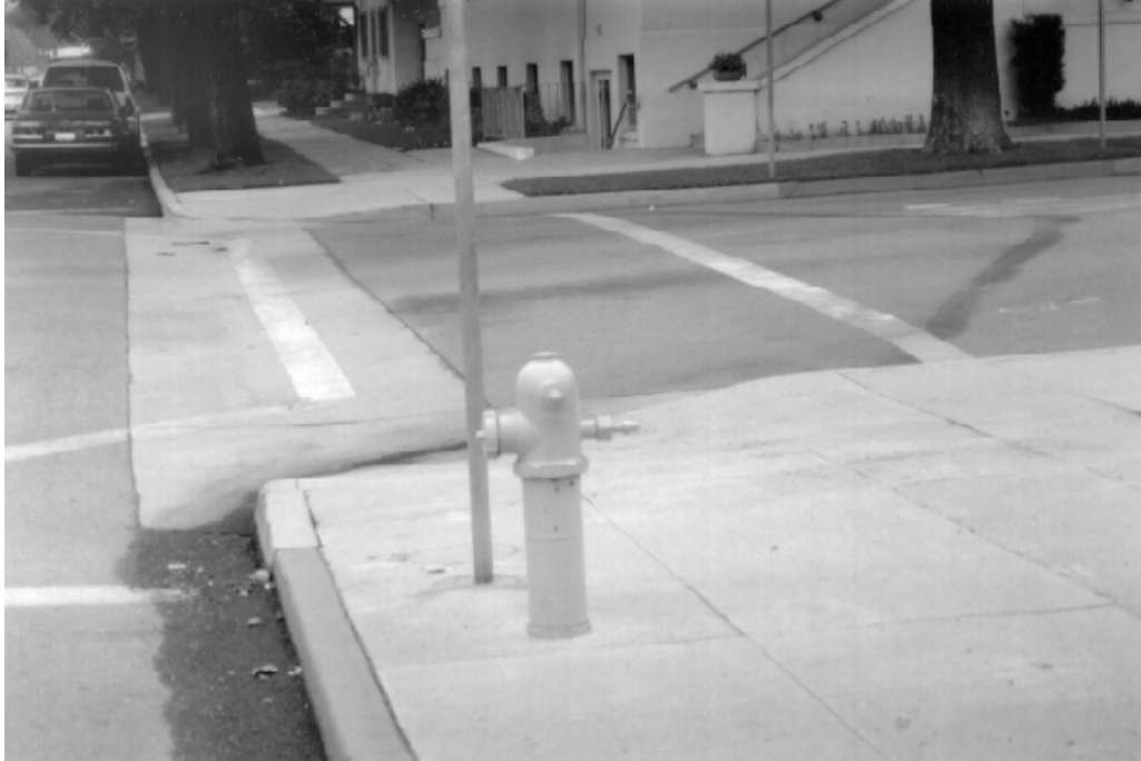
PICTURE 14. TYPICAL FIRE HYDRANT. THE SAFETY ELEMENT REGARDS THE APPROPRIATE PLACEMENT OF FIRE HYDRANTS AND RELATED INFRASTRUCTURE AS WELL AS ADEQUATE FIRE FLOW PRESSURE AS ESSENTIAL STRATEGIES IN MINIMIZING POSSIBLE FIRES.
