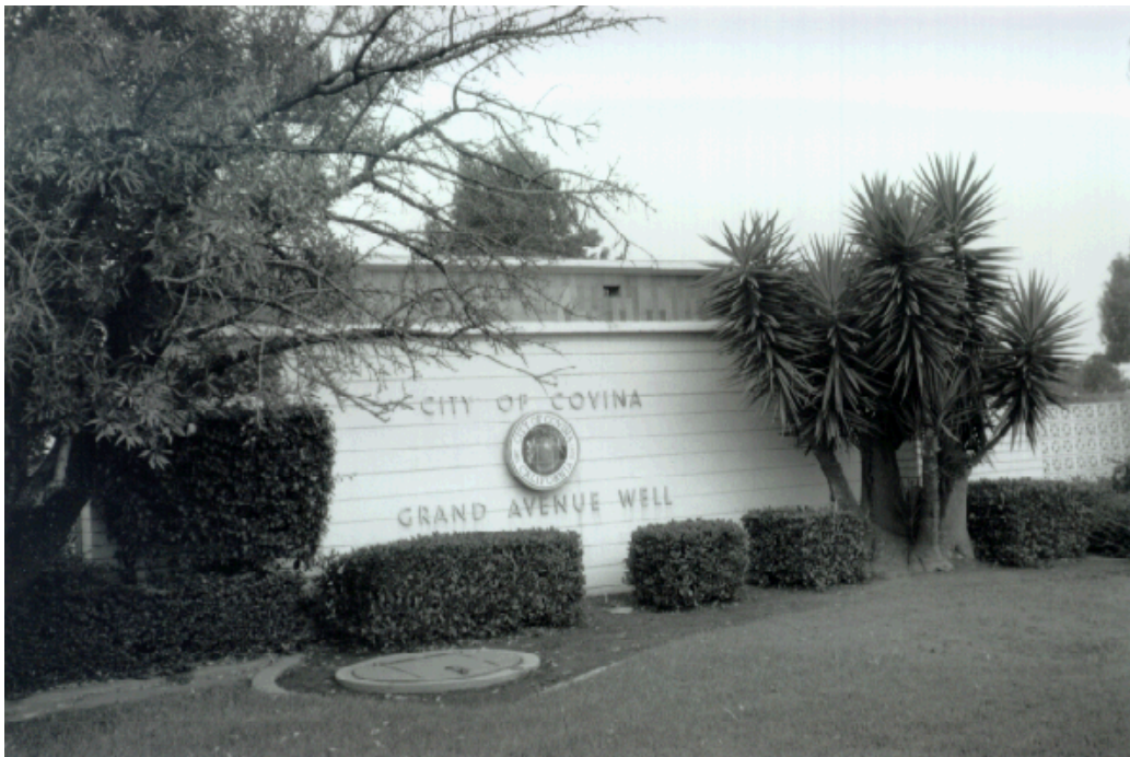
PICTURE 9. COVINA WELL SITE, ON GRAND AVENUE NEAR CYPRESS STREET. WATER EMANATING FROM UNDERGROUND SOURCES, WHICH IS USED FOR ALL PURPOSES IN THE COMMUNITY, WILL CONTINUE TO BE TREATED AND MONITORED TO ENSURE THAT WATER QUALITY STANDARDS ARE MET.
