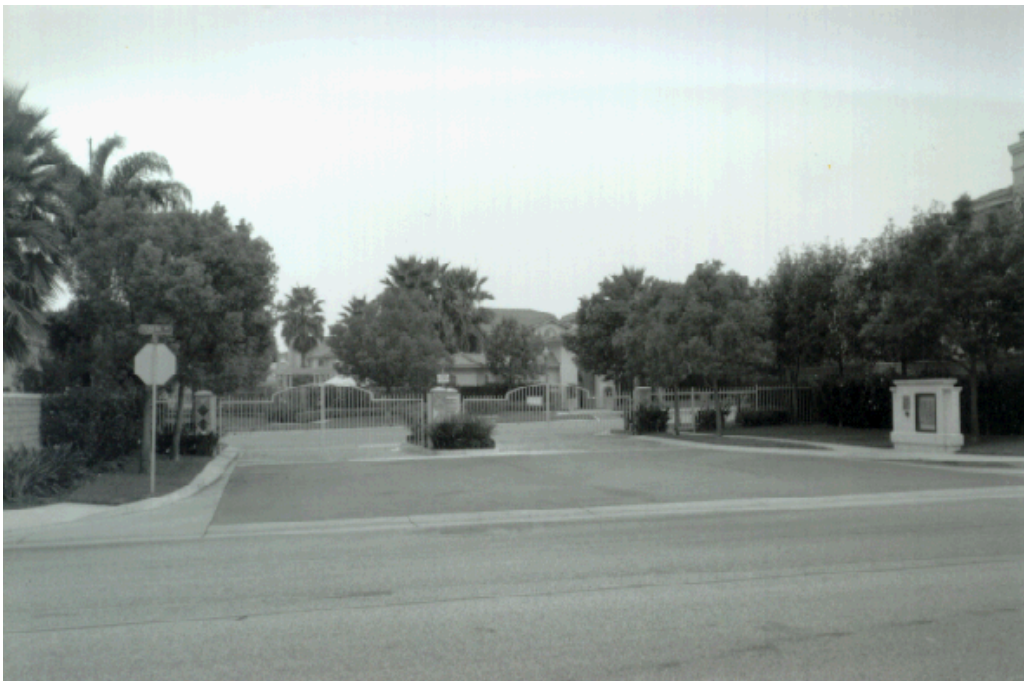
PICTURE 1. MAIN ENTRANCE TO COVINA CLASSICS SINGLE-FAMILY DETACHED AND ATTACHED HOUSING DEVELOPMENT, NEAR BARRANCA AVENUE AND CIENEGA STREET. SOME OF THE NEWER HOUSING PROJECTS IN THE COMMUNITY ARE GATED SUBDIVISIONS.
