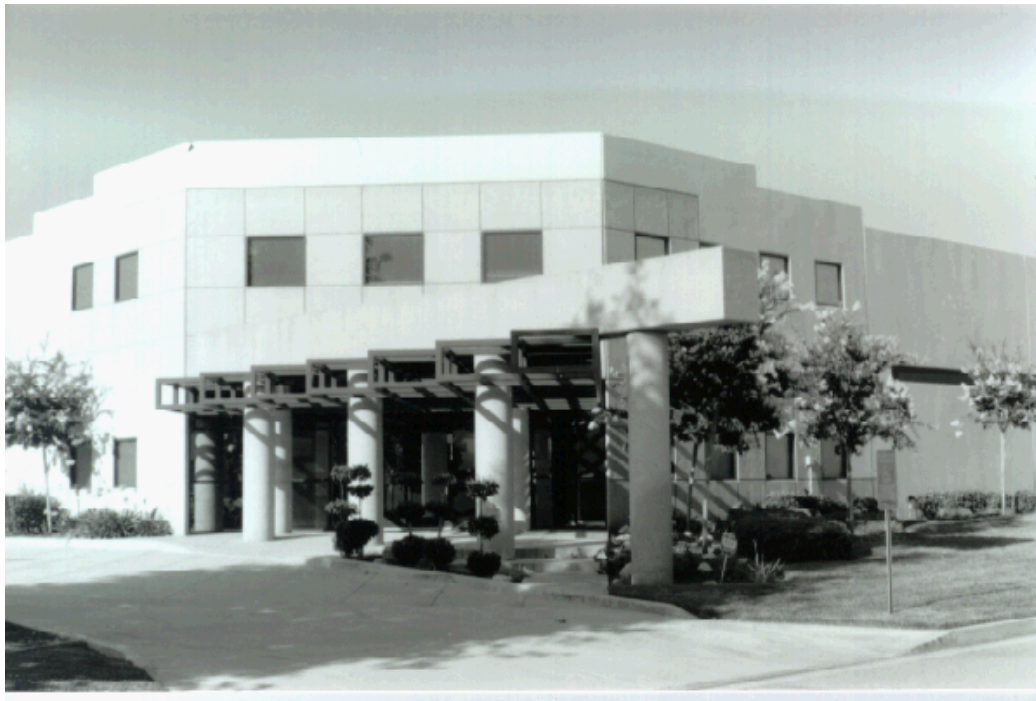
PICTURE 2. TYPICAL INDUSTRIAL BUILDING IN ARROW-GRAND BUSINESS PARK, NEAR GRAND AVENUE AND ARROW HIGHWAY. CURRENT STRUCTURE-RELATED CODES FURTHER GUARANTEE THAT LIGHT MANUFACTURING AND OTHER BUILDINGS THAT ARE IMPORTANT TO COVINA ARE SAFE AND FUNCTIONAL.
