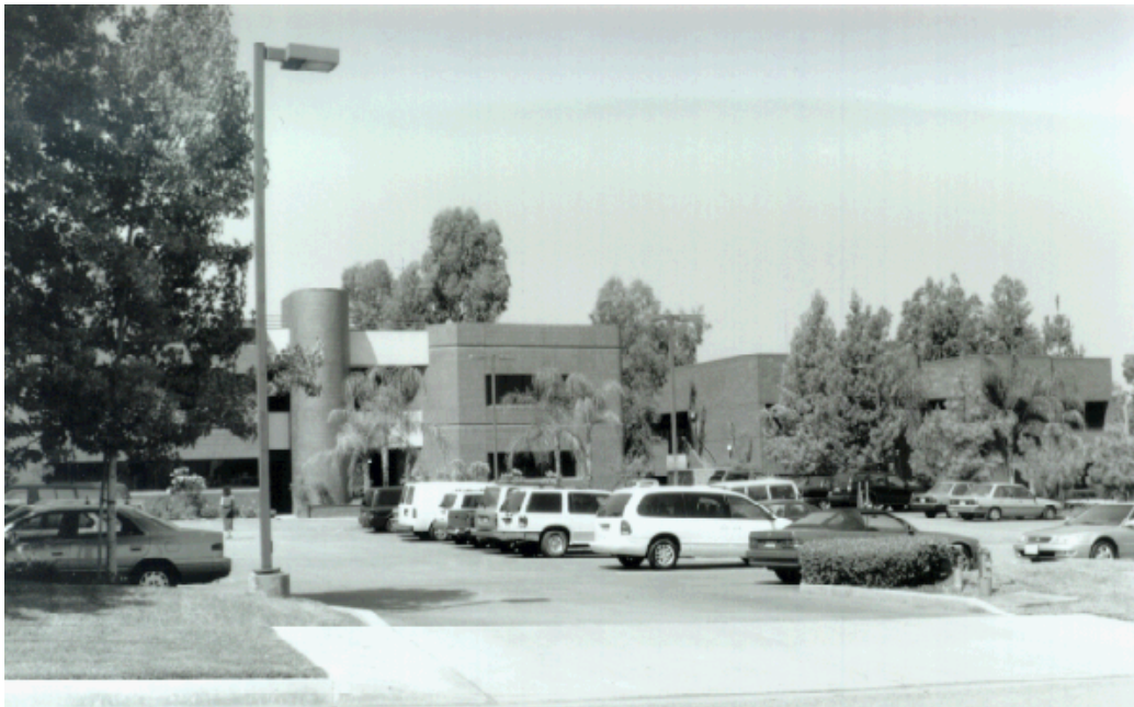
PICTURE 14. OFFICE BUILDINGS IN VILLAGE OAKS OFFICE PARK, NEAR HOLT AVENUE AND SAN BERNARDINO FREEWAY. BESIDES HAVING VARIOUS DWELLING UNIT TYPES, COVINA POSSESSES MANY EMPLOYMENT FACILITIES AND ACTUALLY HAS ABOUT THE SAME DAYTIME AND NIGHTTIME ADULT POPULATIONS.
