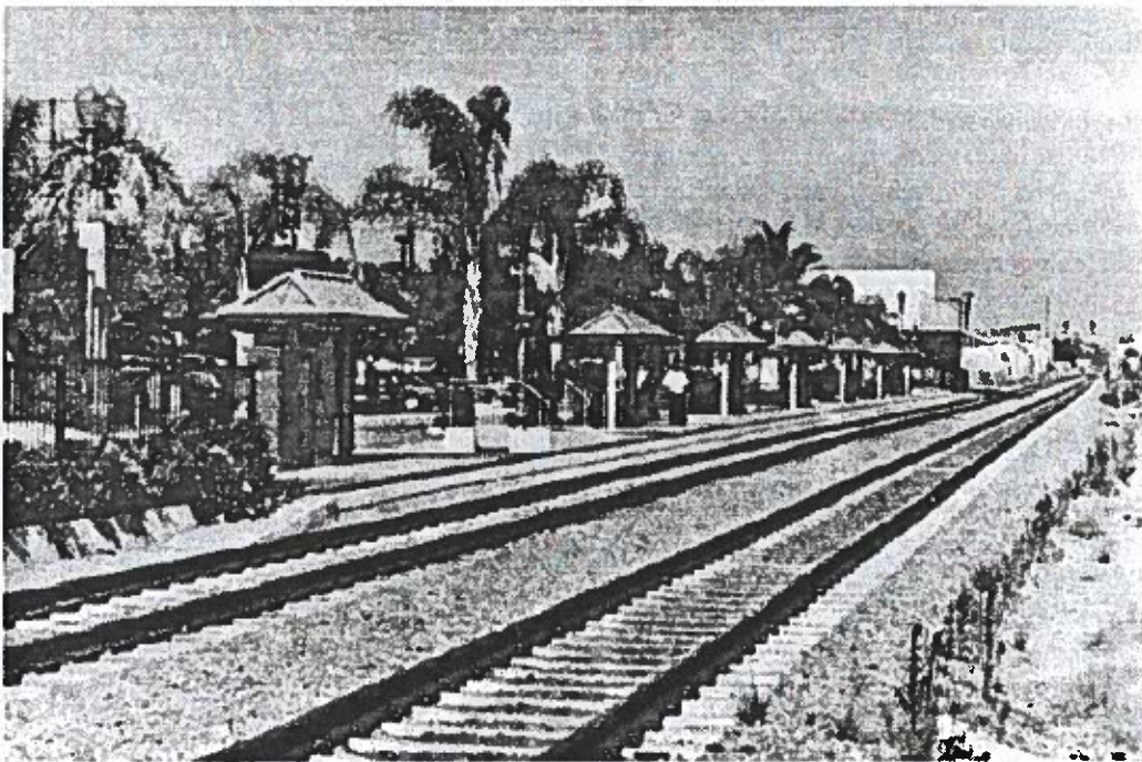
PICTURE 18. COVINA METROLINK COMMUTER RAIL STATION ON CITRUS AVENUE IN NORTHERN PORTION OF DOWNTOWN. GENERAL PLAN POLICY PROMOTES THE LINKING OF THE METROLINK STATION TO THE DOWNTOWN AND OTHER AREAS TO ELIMINATE MANY LONG DISTANCE VEHICULAR TRIPS, THUS REDUCING AIR POLLUTION.
