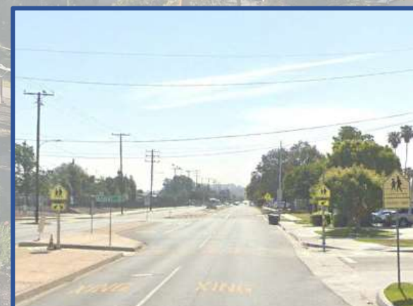
Midblock on Rowland Avenue Pedestrian crossing signage in a school zone with limited visibility of the specific crosswalk location due to faded pavement markings.
