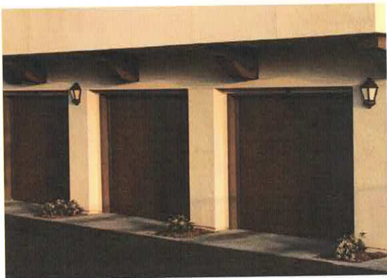
Brackets support cantilever over paneled garage doors
