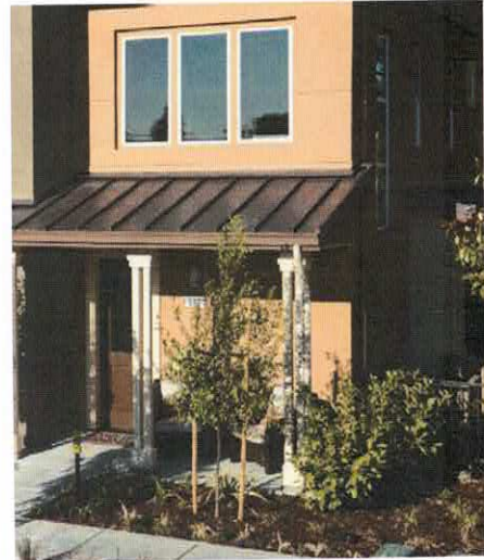
Entry enhanced through awning, front door color application and landscaping
