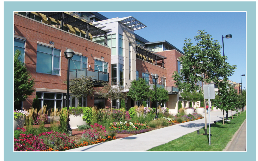
Landscaping softens the appearance of a building along a street
