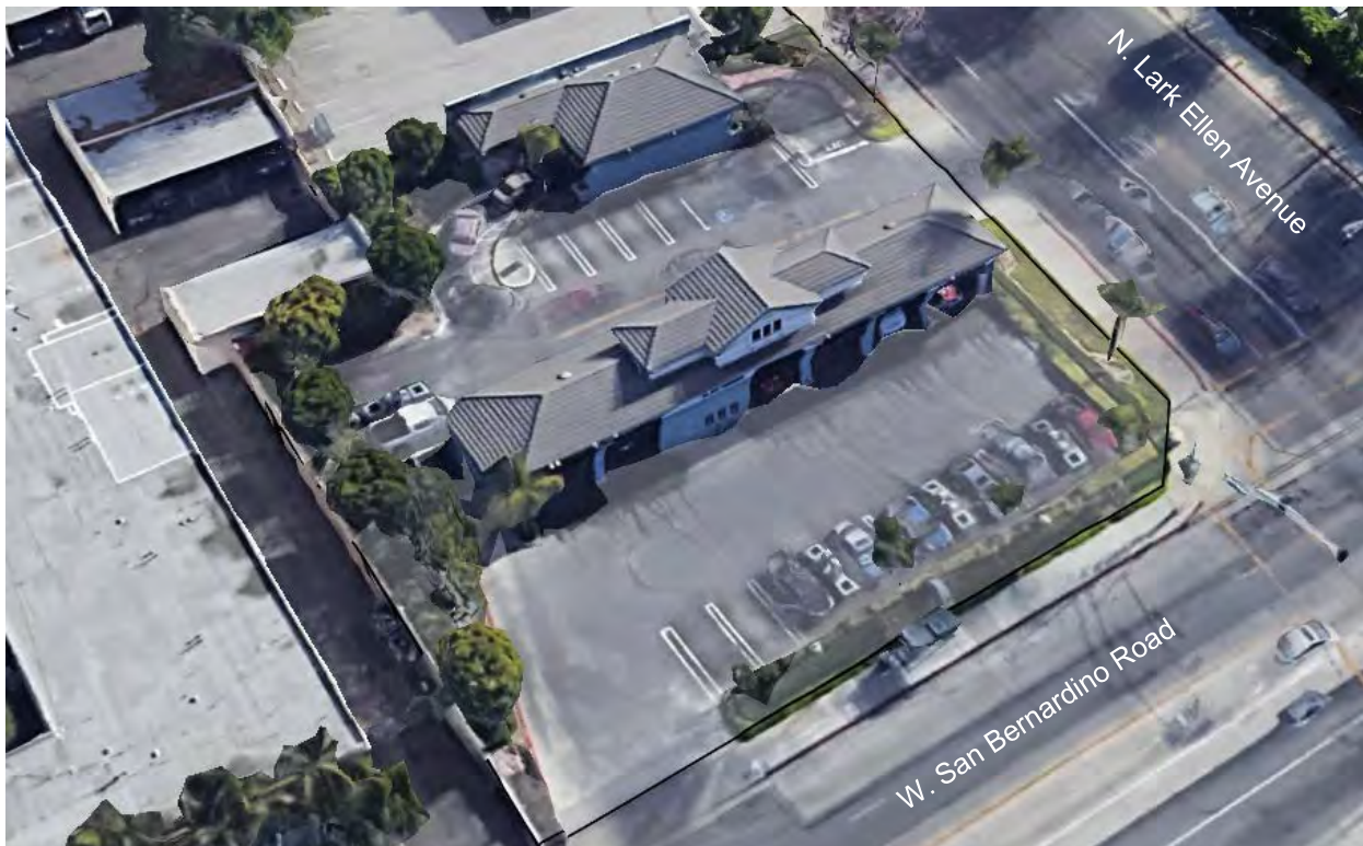
Figure 11. View of parcel (APN:8434-0126-033) which is currently in use as a self-service car wash.
