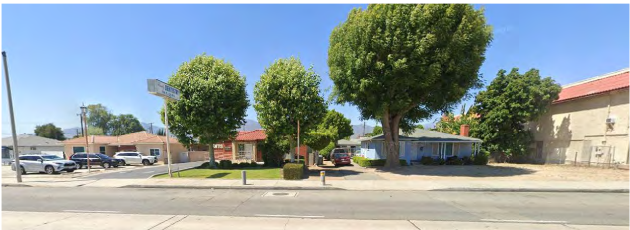
Figure 3. View from W San Bernardino Road facing north.
