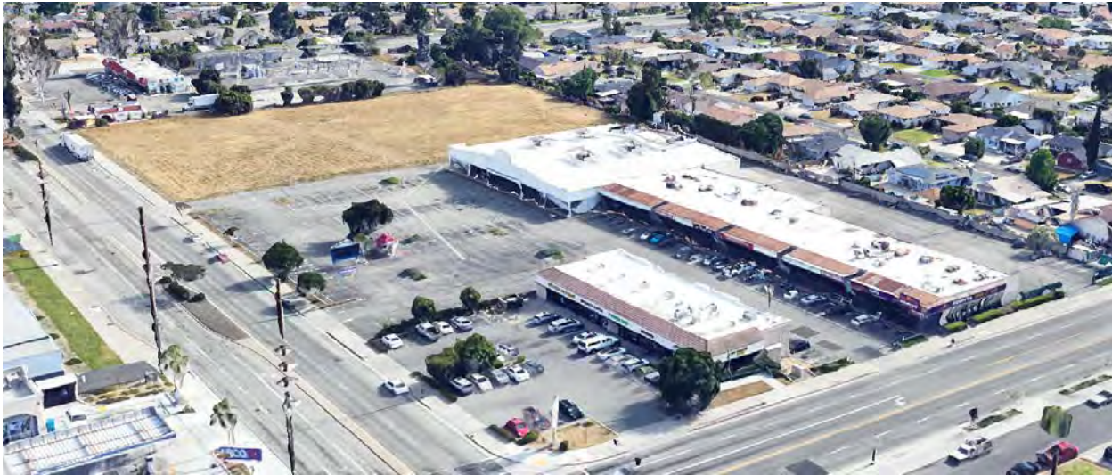
Figure 12. North East Birds Eye View of 4 Parcels in Opportunity Area "M" , on the corner of N. Vincent Ave and W San Bernardino Rd.
