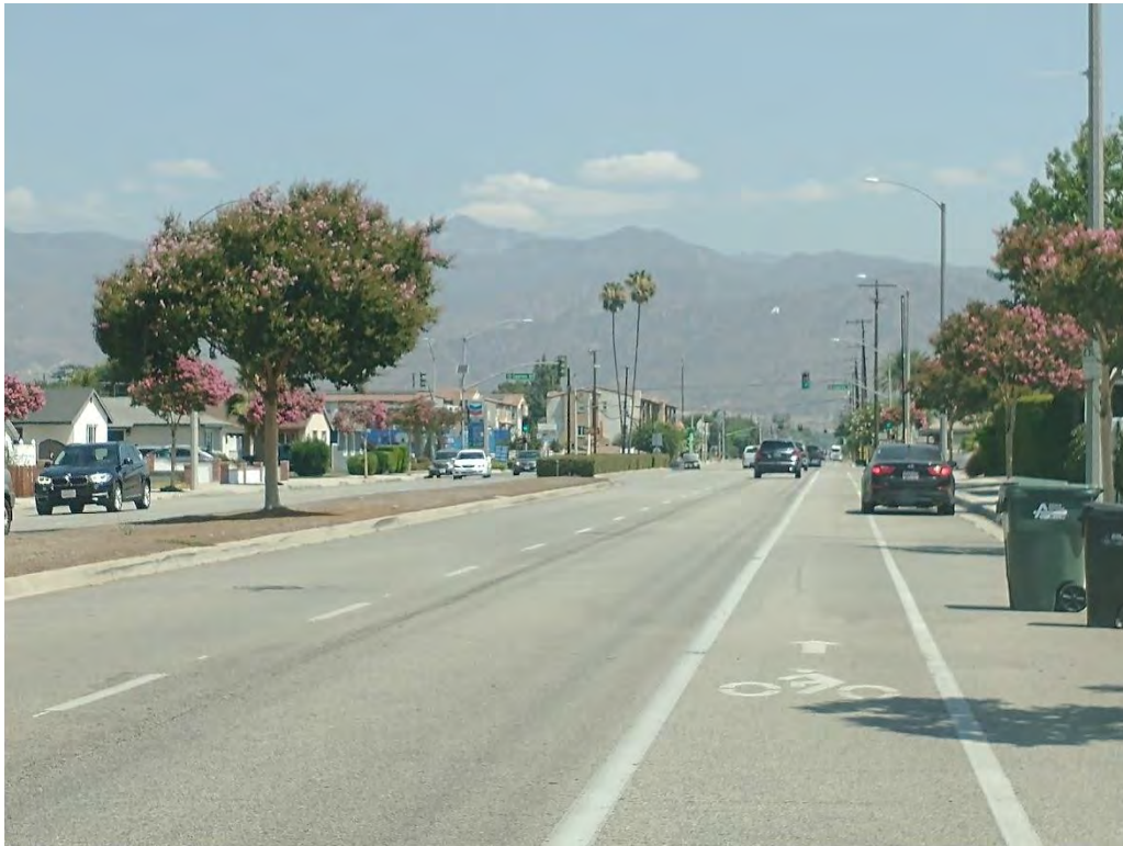
Figure 9 Bike Lane on Citrus Avenue North of Cypress Street
