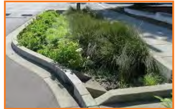
Curb extensions shorten pedestrian crossing distances, slow vehicle turning movements, and can be designed for placemaking or green infrastructure.
