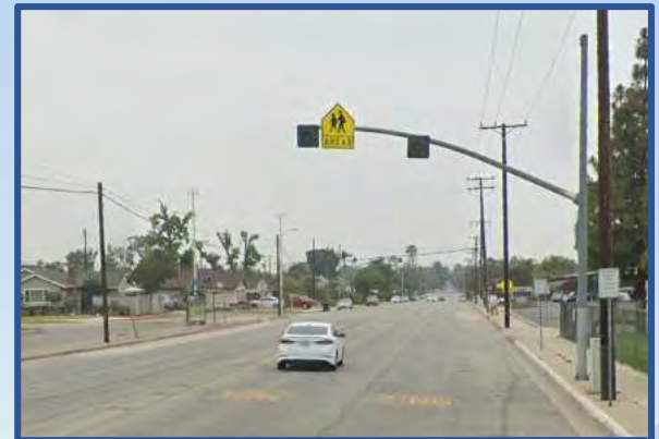
Puente Street near Sierra Middle School Pedestrian flashers ahead of an unsignalized crosswalk. Limited visibility of the specific crosswalk location due to faded pavement markings.
