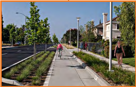
Transformation of Rosemead Boulevard in Temple City created a protected bicycle lane and green infrastructure from excess roadway capacity.
