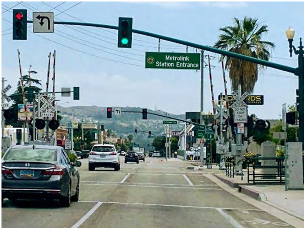
Figure 7 Access to Metrolink Station, Covina
