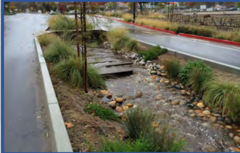
Center medians can be redesigned to provide natural habitat, placemaking, and green stormwater infrastructure.
