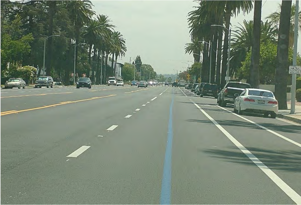
Figure 11 Bike Lane on Badillo Street (East of Hollenbeck) with Parking
