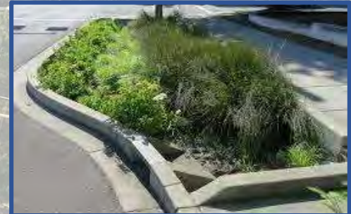
Curb extensions can be added to shorten pedestrian crossing distances, slow vehicle turning movements, and provide green infrastructure.
